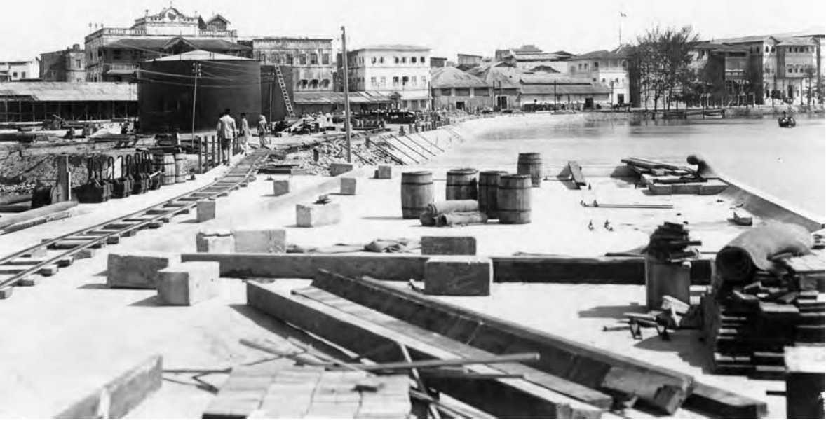
28. Harbor works: new port construction, late 1920s, in the wake of numerous failed plans, prolonged delays, and cost overruns. The Nasur Nurmohamed Dispensary can be seen behind the tank on the left. Zanzibar National Archives.
