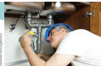
A member of a plumbing LLC.
