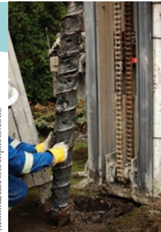
A water well-drilling system.
