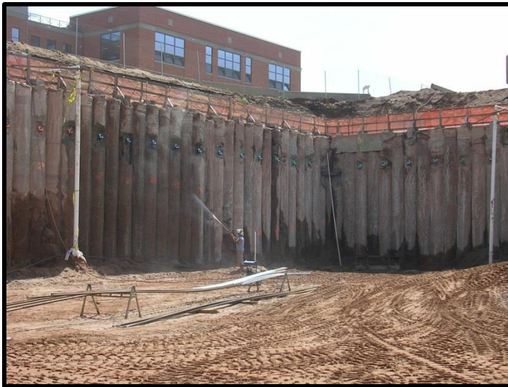
Sheet Pile in basement
