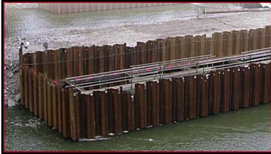
Sheet Piles in Waterfront structure
