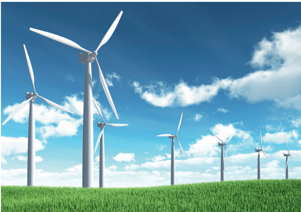
Figure 5.4 Wind energy farm generators.
