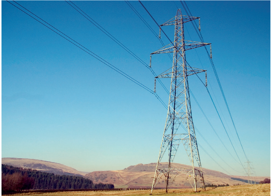
Figure 3.28 Transmission line steel pylon.
