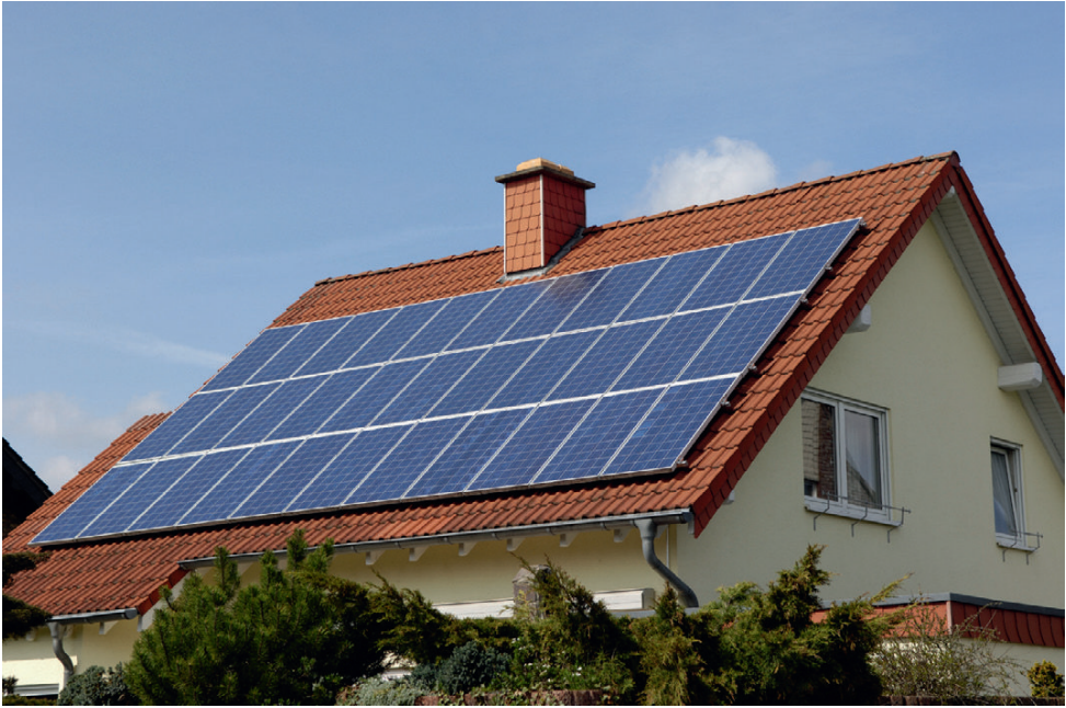
Figure 5.1 Photograph of PV system in a domestic situation.
