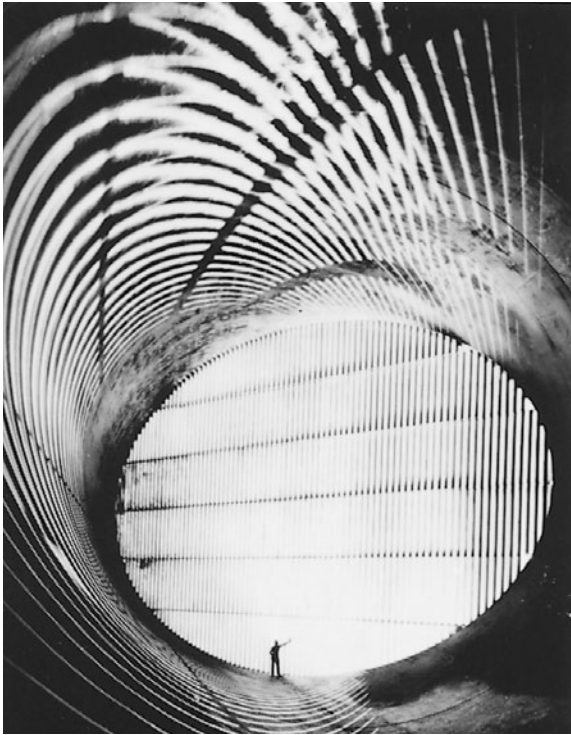
Figure 5.7 This giant air passage houses a massive set of stationary guide vanes in one elbow of a wind tunnel which force the air to make a right angle smoothly. (Courtesy of the National Aeronautics and Space Administration.)
