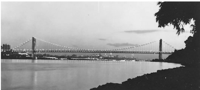
Figure 1.11 The George Washington Bridge. (Courtesy of the Port Authority of New York and New Jersey.)
