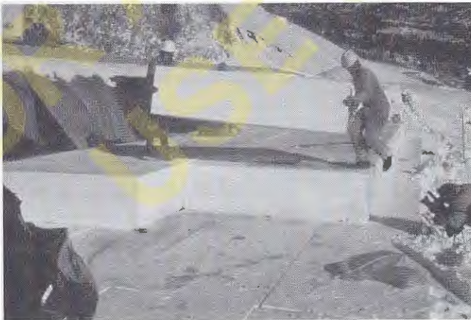
Figure 6.39 Geofoam blocks being placed to produce a lightweight fill for a highway in Colorado. (BASF Corporation)
