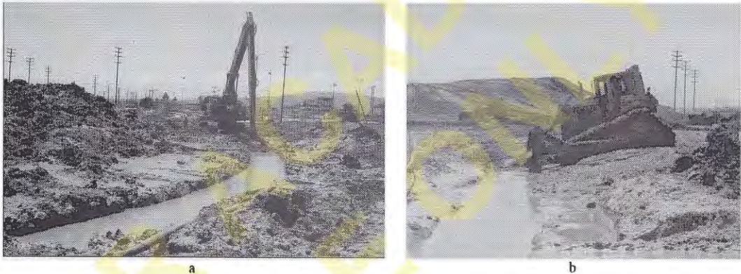
Figure 8.32 A slurry trench barrier under construction: a) An excavator is digging the 20 m (65 ft) deep trench through a slurry, b) then a bulldozer pushes in a clayey backfill.
