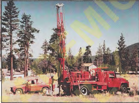
▼ Plate J Drilling an exploratory boring
