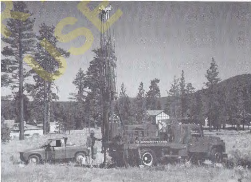
Figure 3.5 Truck-mounted drill rig.
