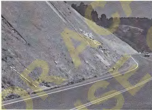
Figure 14.41 A series of horizontal drains in a cut slope along a highway. The close-up view shows one of the drains exiting the slope and discharging into a swale. This drain has a slow but continuous flow, as evidenced by an accumulation of algae at its discharge point.
