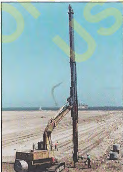
▼ Plate O Wick drains being installed ( American Wick Drain Corporation )
