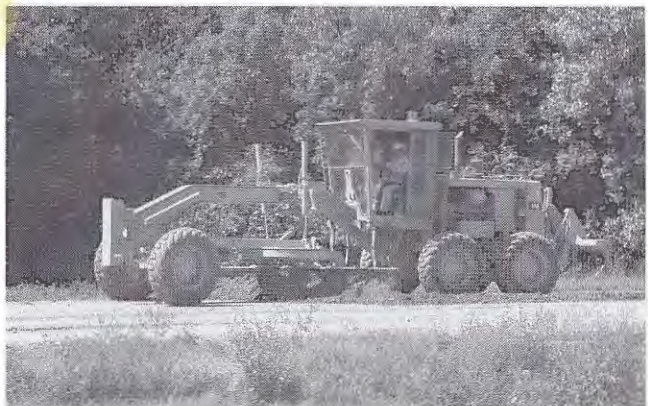
Figure 6.24 A motor grader fine grading a highway subgrade. (Caterpillar Inc.)
