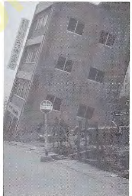
Figure 20.10 The soils below this building in Niigata, Japan, liquefied during the 1964 earthquake, causing settlement and bearing capacity failures. (Earthquake Engineering Research Center Library, University of California, Berkeley, Steinbrugge Collection)
