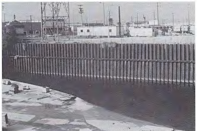
Figure 16.23 A sheet pile wall.
