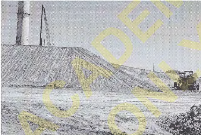
Figure 19.1 This surcharge fill will remain in place until the underlying soils have settled. The smokestack and crane in the background are located behind the fill.
