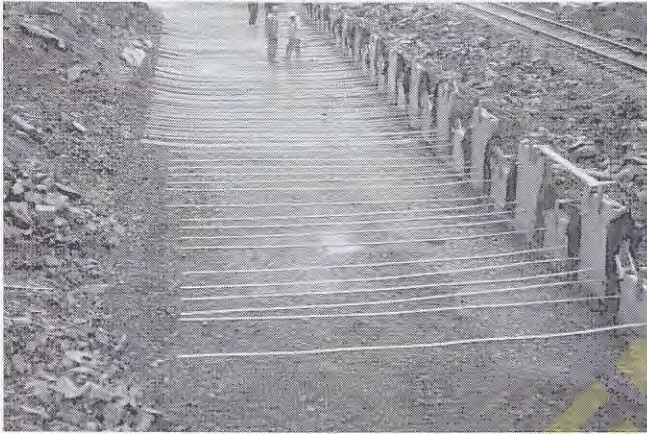
Figure 16.26 Reinforced earth walls consist of precast concrete facing panels and steel or polymer reinforcing strips that extend into the retained soil. This wall is under construction (The Reinforced Earth Company).
