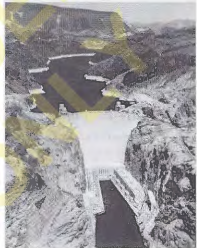
Figure 15.2 Hoover Dam on the Colorado River at the Nevada–Arizona border. This is a concrete arch dam (U.S. Bureau of Reclamation).
