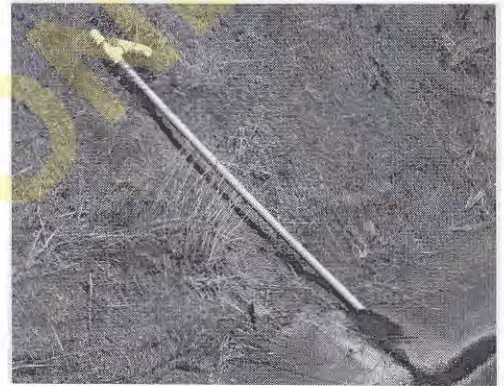
Figure 14.41 A series of horizontal drains in a cut slope along a highway. The close-up view shows one of the drains exiting the slope and discharging into a swale. This drain has a slow but continuous flow, as evidenced by an accumulation of algae at its discharge point.
