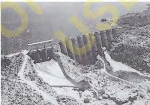
Figure 15.3 Bartlett Dam on the Verde River in Arizona is a concrete buttress dam (U.S. Bureau of Reclamation).
