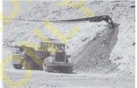
Figure 6.17 Use of conveyor belts to transport soil to the Seven Oaks Dam in California. These belts move soil about 3 km (2 mi) from the borrow site to the dam, then drop it at a convenient location. The loader places it in large dump trucks that haul it a short distance to the construction site.
