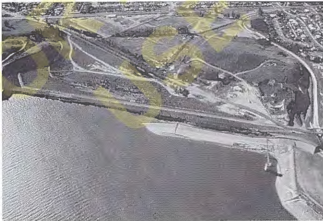
Figure 20.8 Lower San Fernando Dam. The soils inside this earth dam liquefied during the 1971 Sylmar Earthquake in California. The dam was constructed by hydraulic filling (see Chapters 6 and 15), and thus contained loose, saturated, sandy soils prone to liquefaction. The left portion of the dam slid into the reservoir, leaving only 1.5 m of freeboard. The failure of this dam prompted the reconstruction or replacement of several other dams that also had been built using hydraulic filling.
