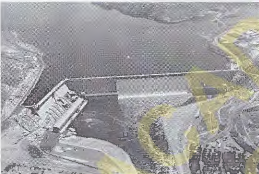
Figure 15.1 Grand Coulee Dam on the Columbia River in Washington. This is one of the largest concrete gravity dams in the world (U.S. Bureau of Reclamation).
