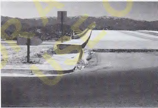
Figure 11.2 The approach fills adjacent to this bridge in California have settled. However, the bridge, being supported on pile foundations, has not. Note the abrupt change in grade in the sidewalk, and the asphalt patch between the two signs. This photograph was taken about twelve years after the bridge was built.
