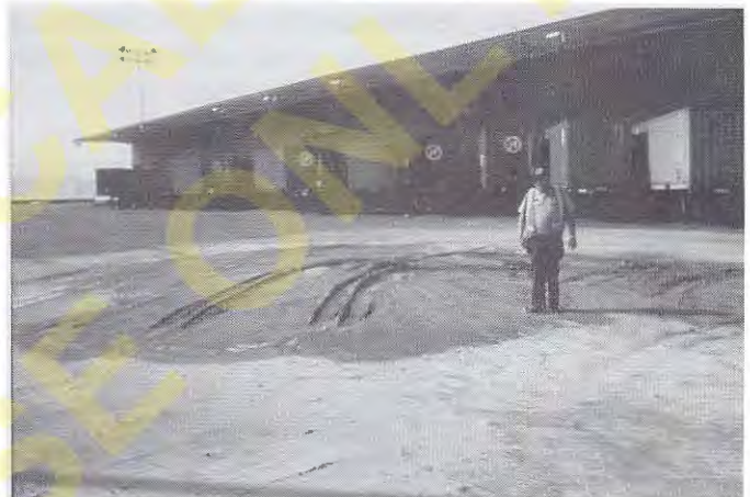
Figure 20.6 Sand boil at truck terminal in Port of Oakland, California, produced by the 1989 Loma Prieta Earthquake. (Earthquake Engineering Research Center Library, University of California, Berkeley, Steinbrugge Collection)
